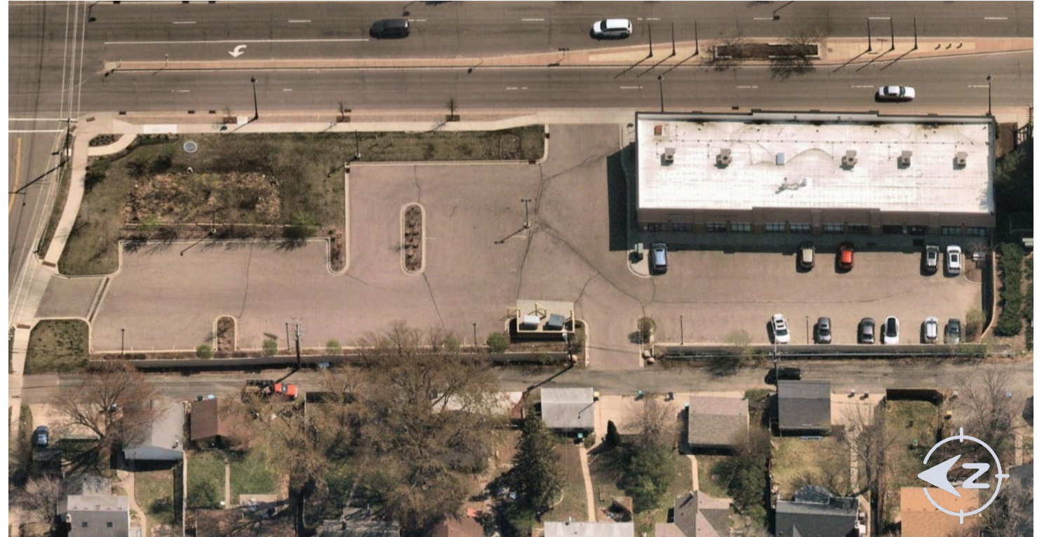
Parking lot was re-stripped in 2024
