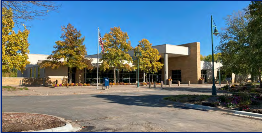
Eagan Community Center in Eagan. Source: LOCi Consulting LLC
